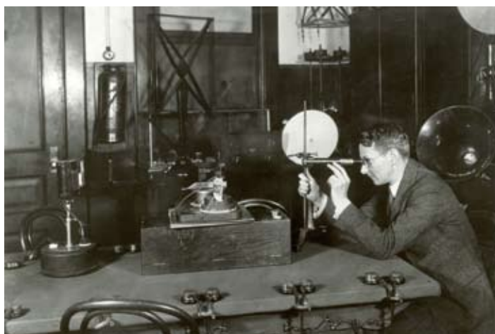
Alexander McLean Nicolson in The Western Electric research department (AT&T) c. 1920. Nicolson observes crystal motion on the box in the table with a Fabre Perot interferometer. The white disc just over Nicolson's hands is the paper cone of a piezoelectric crystal driven load-speaker of his design. From AT&T archive.
