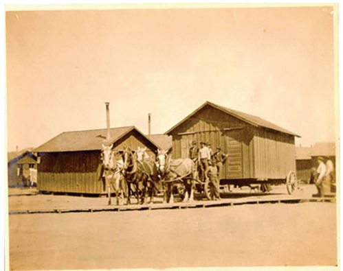
Figure 2: A San Francisco “Earthquake Cottage” being carted off to its new home ( San Francisco History Center, San Francisco Public Library ).
