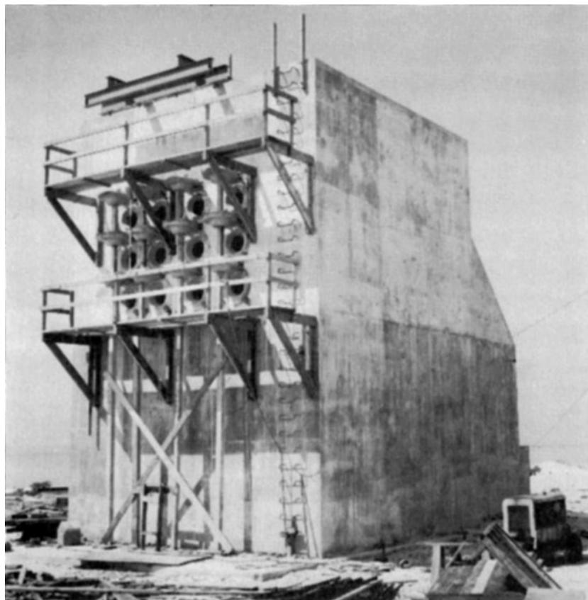
Fig. 18: Berlyn Brixner. Concrete bunker for photographing the first thermonuclear test *Ivy Mike* at Eniwetok Atoll, Marshall Islands. 1952. Source: Brixner 1993: 57.
