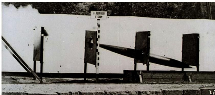
Fig. 25: Albert Londe and Hippolyte Sebert. Photograph from a sequence showing a torpedo's flight through paper screens. c. 1890. Source: IWF Wissen und Medien, Göttingen.
